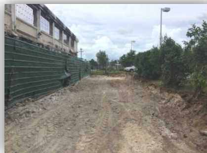
August 8, 2017 – After encroachment was removed
