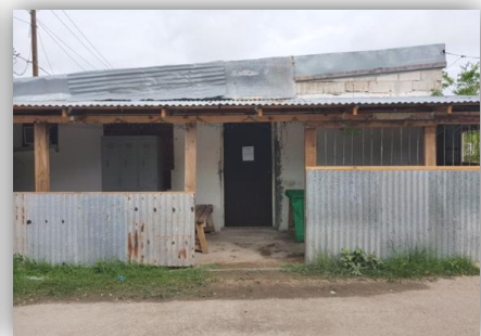
In December 2017, DPL reclaimed this lot which was not in compliance with DPL's regulations
