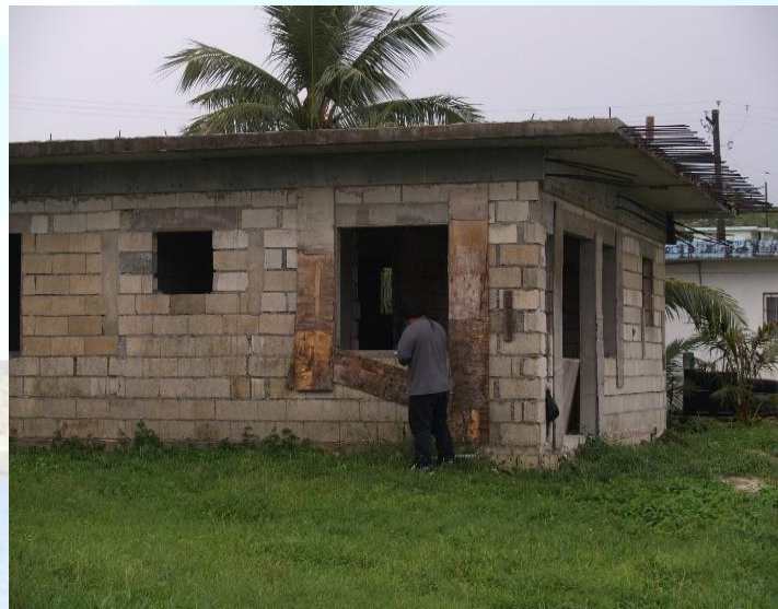
Homestead Site Inspection
